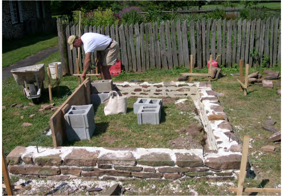
Master stone mason Keith Childs building the foundation for the woodshed
